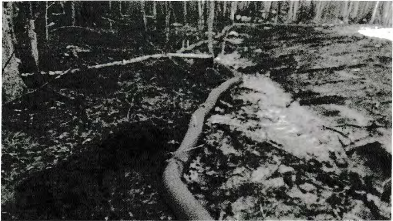
Picture 6-Breach near up to and within outer portions of isolated forested wetland H. Mulched chips and stone placed to prevent erosion.
