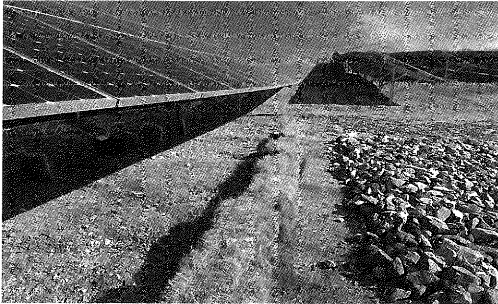
Photo 9: Eastern side of Wetland F, some new erosion control reinforcements:
